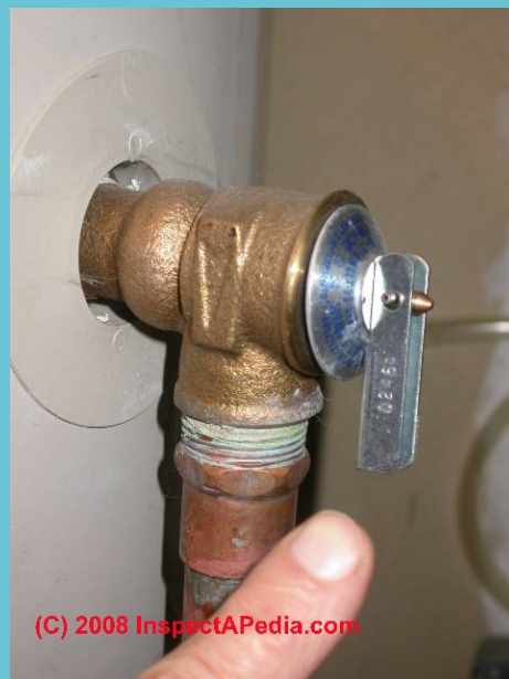
Pressure Reducing Valve
